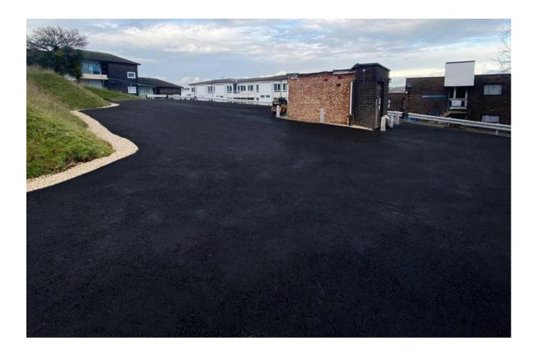
The £50,000 project included levelling the rough ground and removing vegetation before applying a substrate of type 1 aggregate. Tarmac surfacing was laid and marked with parking bay divisions, kerbs and edging established and areas of light-coloured gravel were used to enhance the aesthetic landscaping of the car park. Concrete safety bollards were also installed around an existing utilities hut to complete the well-planned car park design.
