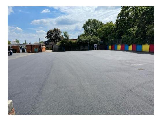
The work covered over three playground areas where the surface had become very brittle, but care was needed to ensure that the surfacing did not extend beyond existing perimeters. This required a high degree of accurate planning. We also installed a new footpath and entry pathway, as well as constructing a new drainage system.
